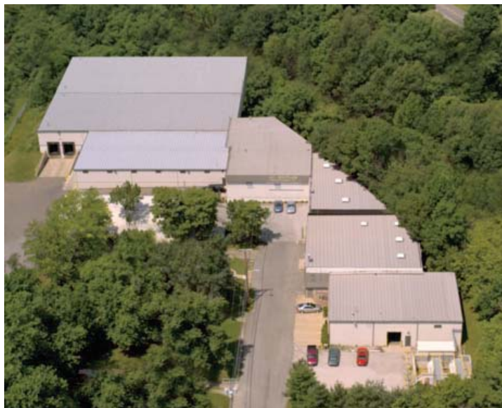
J.C. Whitlam Manufacturing Headquarters consists of more than 100,000 square feet of offices, plant, warehousing and laboratory facilities in northeastern Ohio. Chemical containment tanks, shown above, allow proper storage and quick retrieval.
